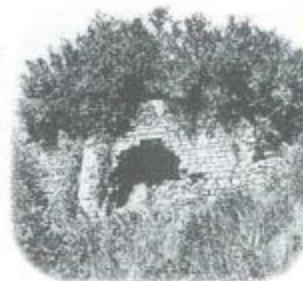
Meilhan tunnel entrance
