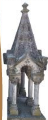
Pinnacle on top of columns at the Meilhan's church
